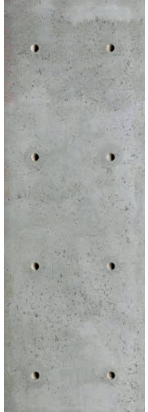
Exposed Concrete Columns (Select Units)
